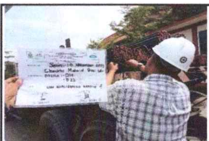
Checklist Materai on site besi beton
